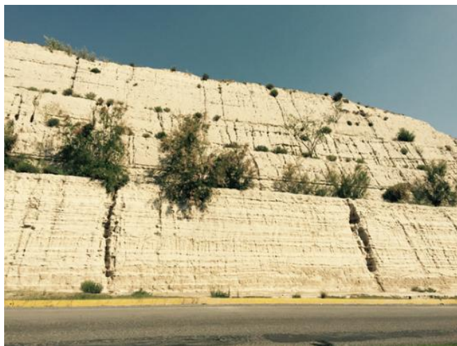
Figure 2. Mine waste material.
